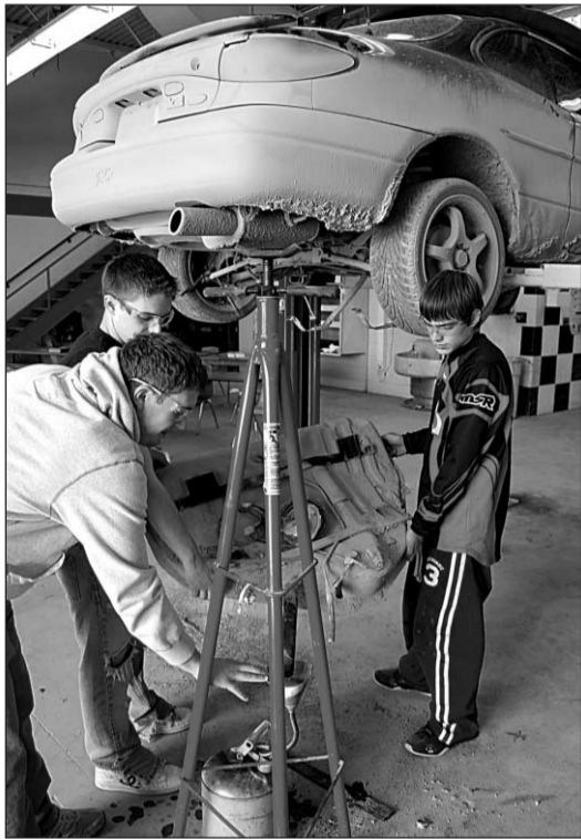
Students in Automotive Technology use their training to maintain their own vehicles. Here Ford Escort owner Robert Roche of Ray Township is assisted by Luke Kujawa of Armada and AJ Leonard of Richmond. Rob's fuel pump failed and they needed to remove the tank to make the repair.
